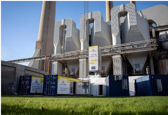
Pilot carbon capture plant at cement plant in Aalborg, Denmark
