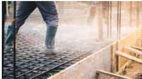
(b): In-situ cast concrete for a road bridge
