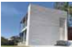
Pre-cast and concrete elements, Couldrey house, Australia
